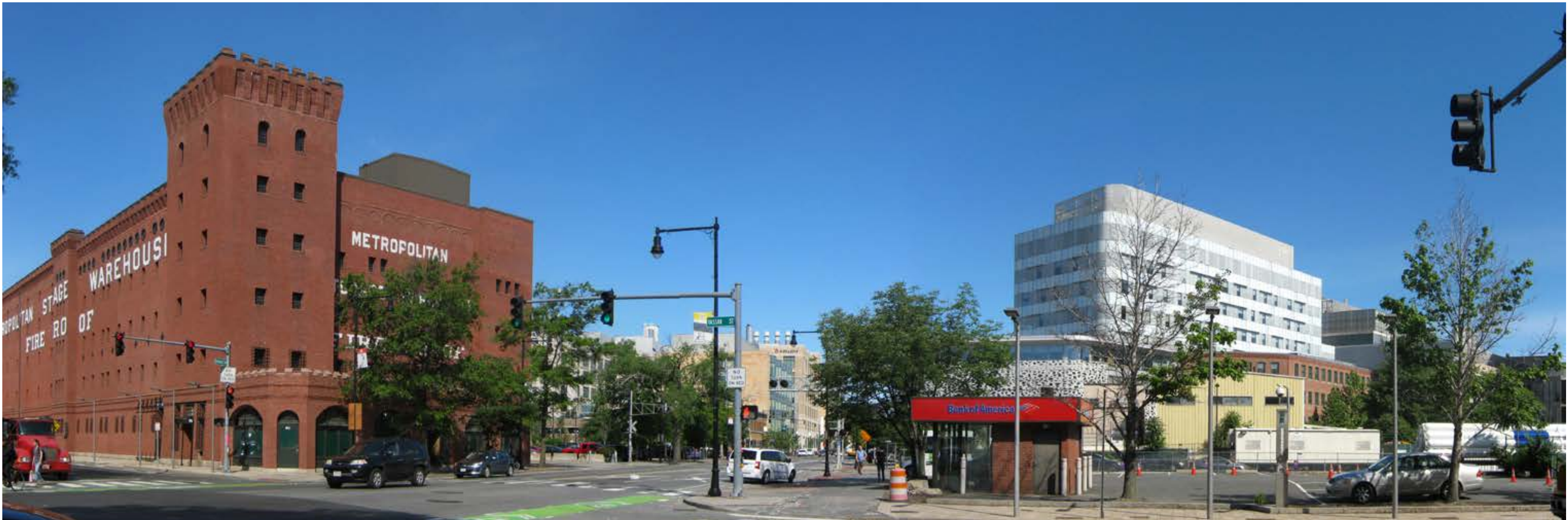
4 Mass. Ave. at Vassar Street.
