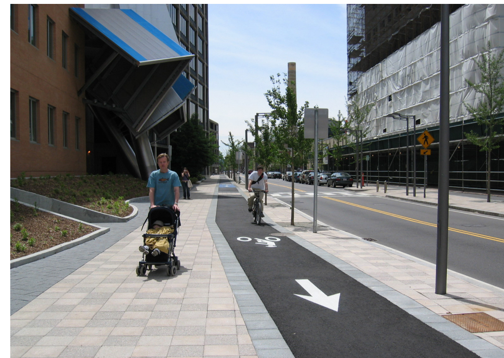
The Vassar Street cycle track separates bicycle, pedestrian, and automobile traffic so that all users feel more comfortable.
