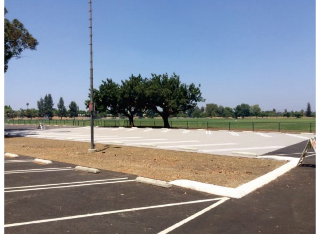
Cool pavement with gray coating is 10 degrees cooler than black asphalt.
