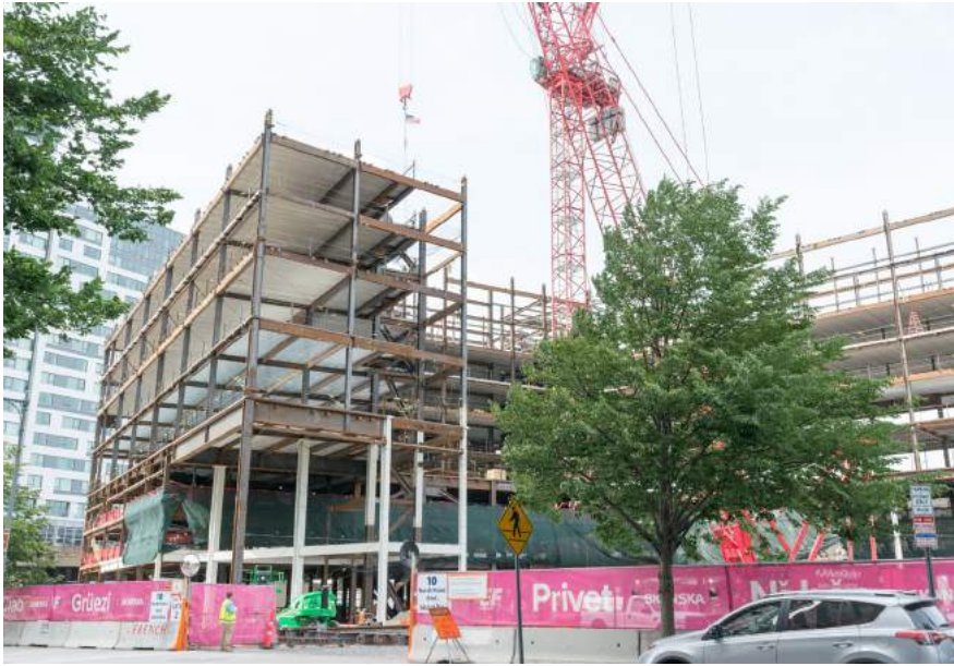
Planned development under construction at North Point/Cambridge Crossing, 2018.
