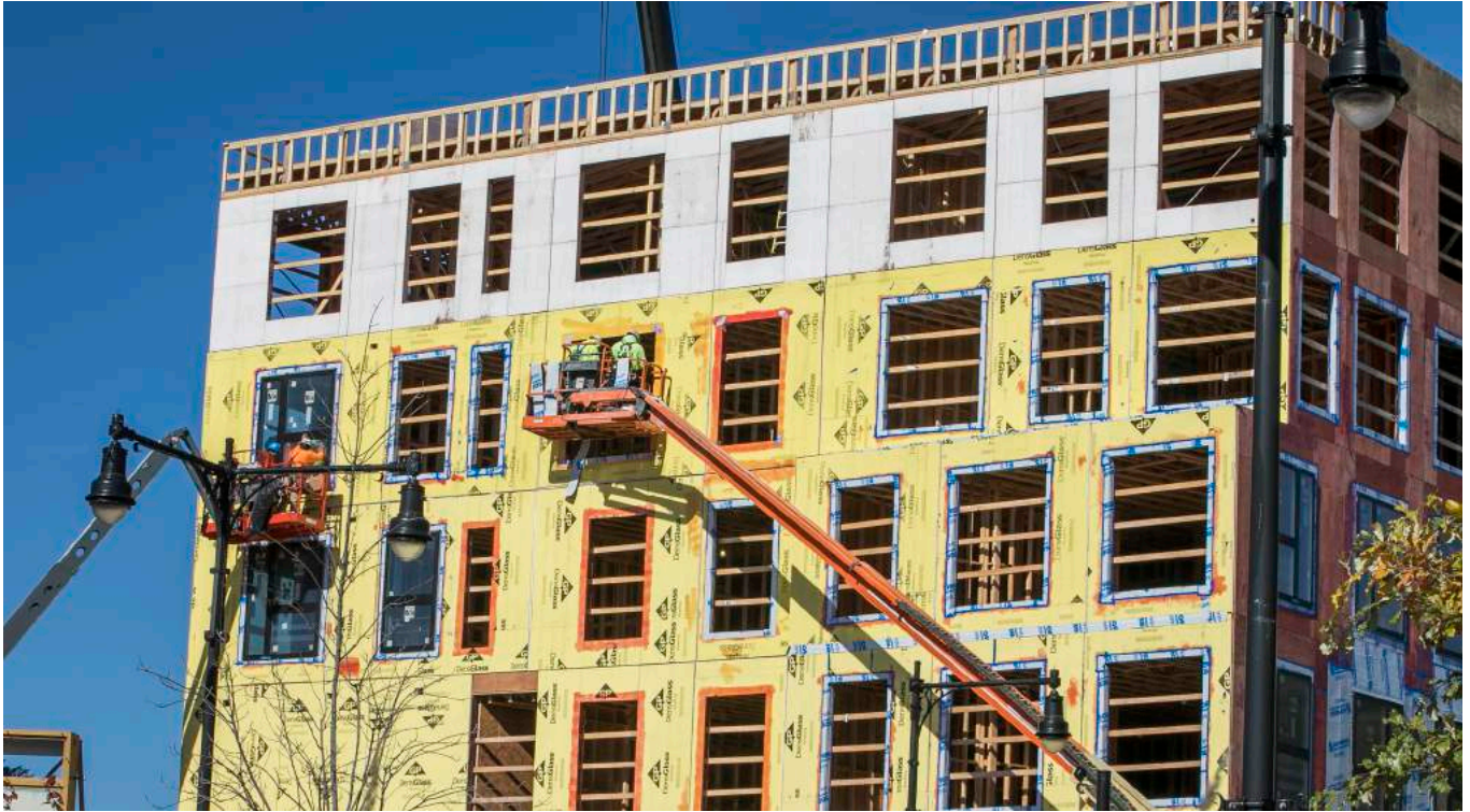
Construction in Cambridge in fall 2018.
